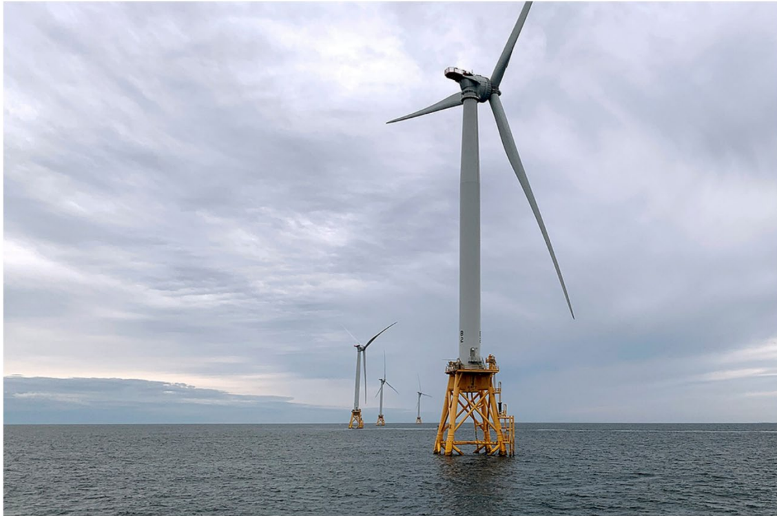
Deepwater Wind's turbines stand in the water off Block Island, R.I. Rodrigue Ngowi/AP Photo
